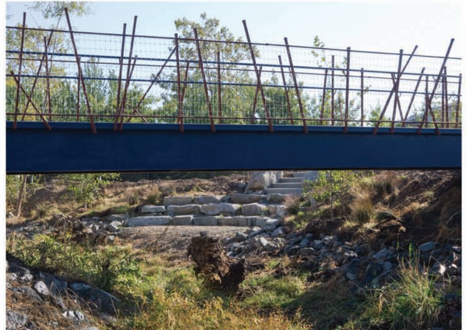
View of Castro Valley Creek and pedestrian bridge made from a converted railroad flatcar. The creekside amphitheatre can be seen in the background.
