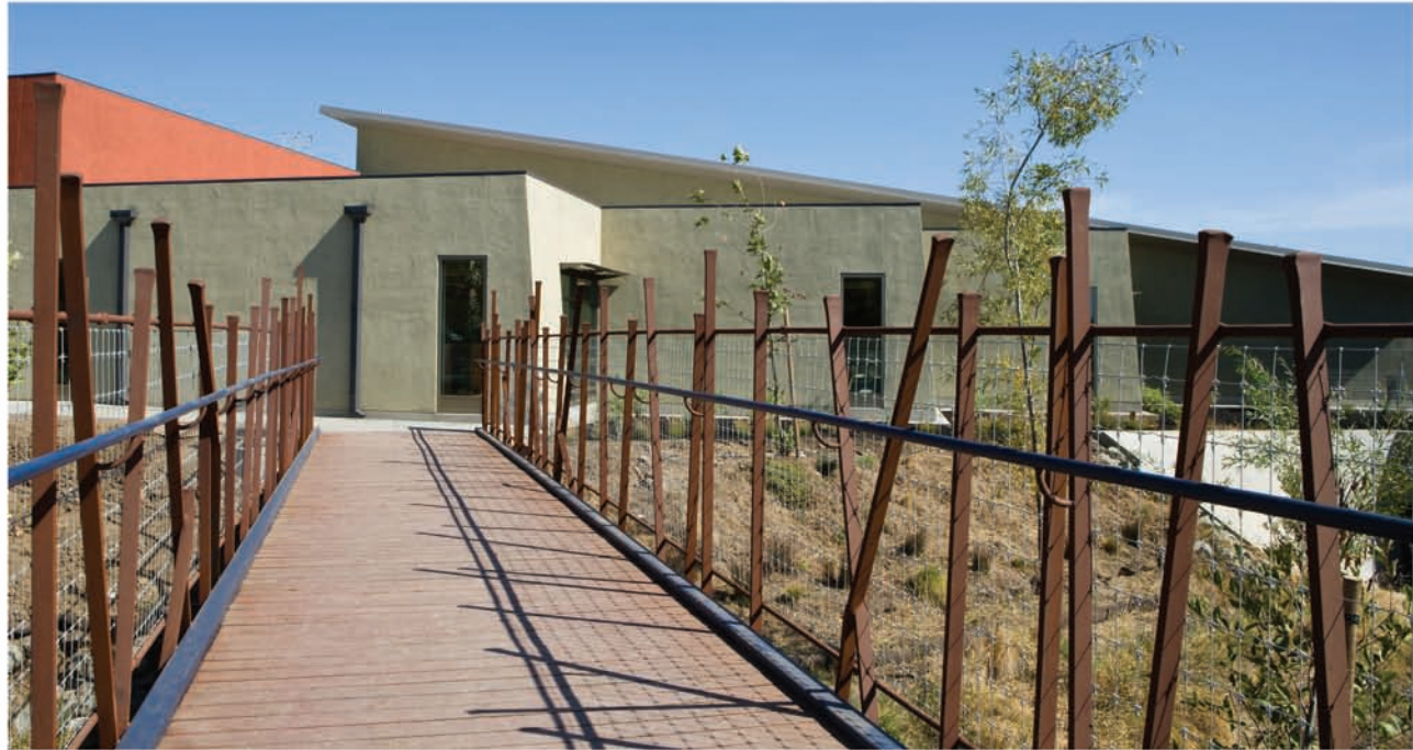
Elevated Fence Project, 2009, Weatherproof steel and galvanized steel, 1200 linear feet of fence and bridge railing
