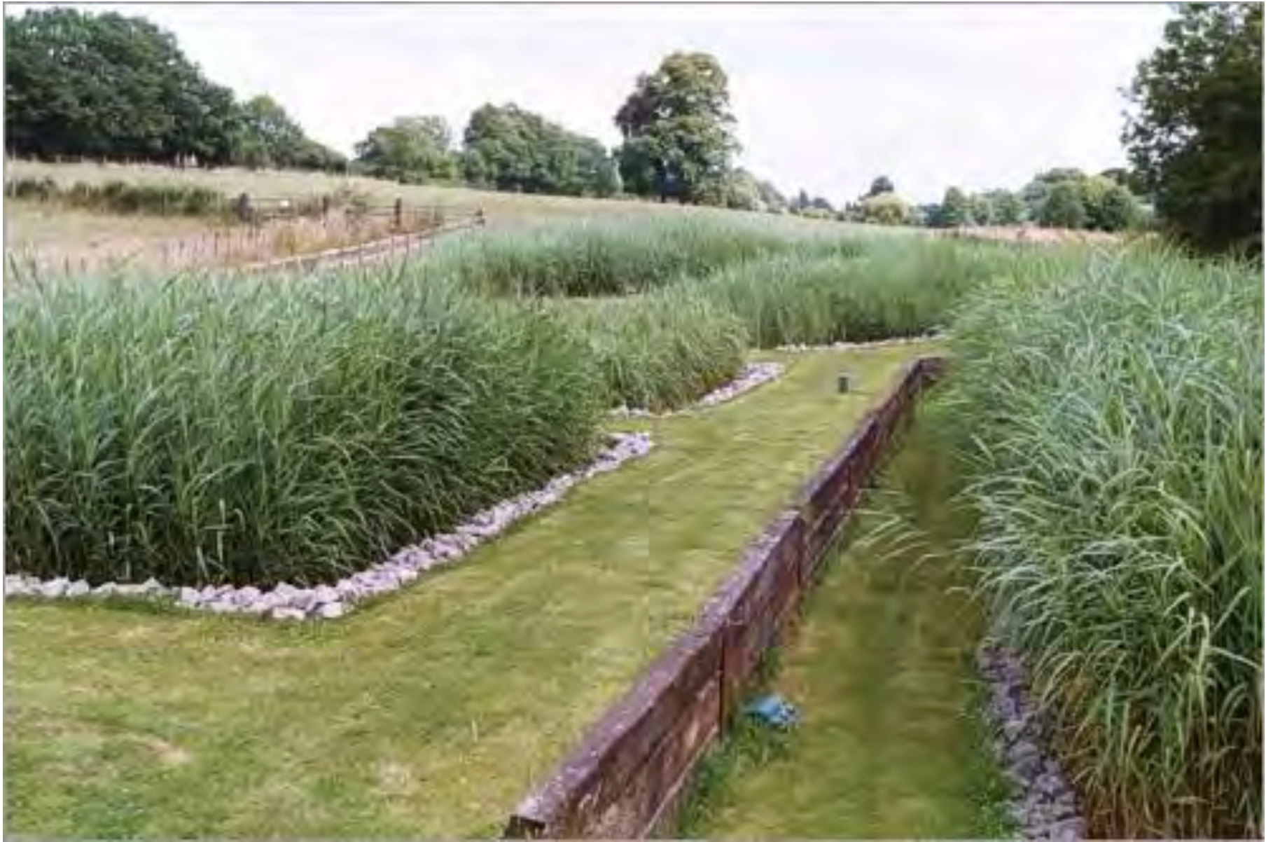
Reed bed Wastewater Wetland - UK
