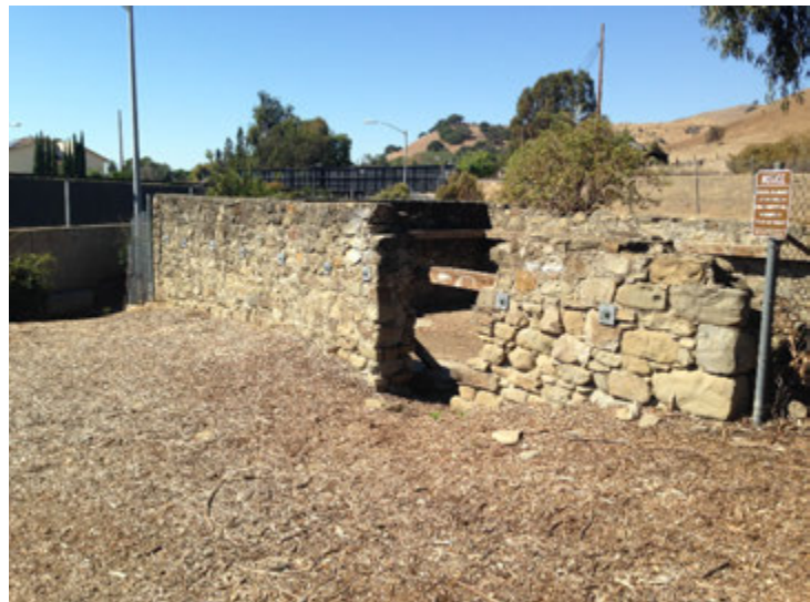
Exposed foundation of the 1856 mill located near the Mission Boulevard.
