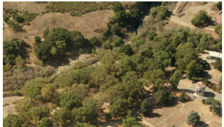
The bridge options to cross the Alameda Creek are both located behind the Sunol Water Temple.
