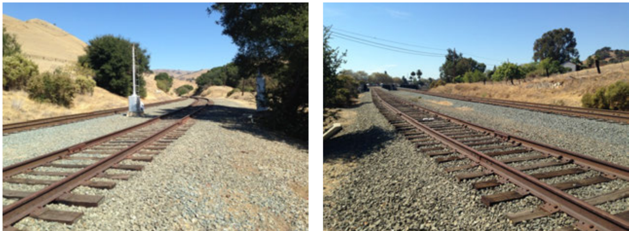
Location of at grade track crossing
