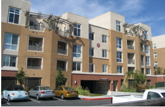
Tuck Under Parking. Parking is located on the ground floor under the units. (Guideline G-1)
