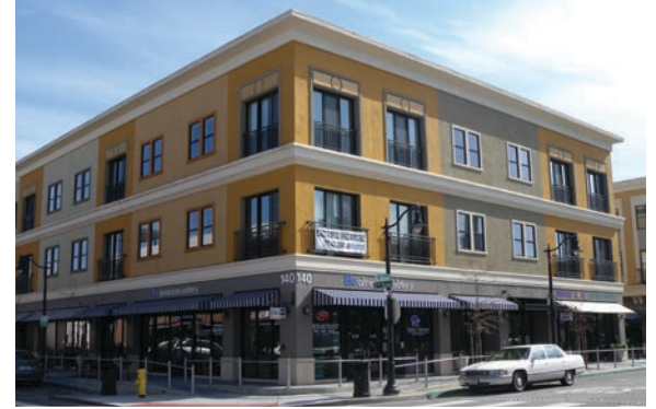
Using different colors on a building facade is not a successful way of providing vertical articulation as it does not create shadow or provide architectural relief. (Guideline E-26 & 27)
