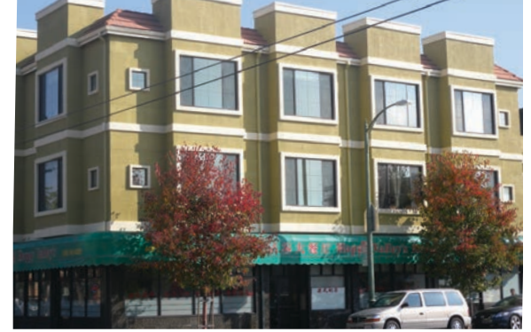
Although this project incorporates several articulation elements such as window trim, belt course, and variable roof forms, the unbalanced facade composition (overly heavy third story), disproportionate windows, non-harmonious roof forms produces an overly bulky building. (Guideline E-26 & 27)
