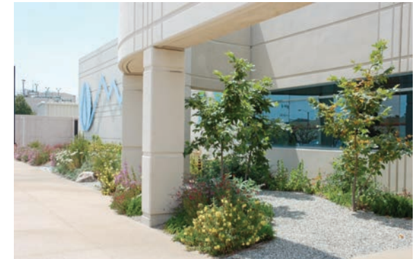
Select landscape materials that are hardy enough to withstand close contact with pedestrians and vehicles and that cover bare dirt once fully grown. (Guideline J-13)
