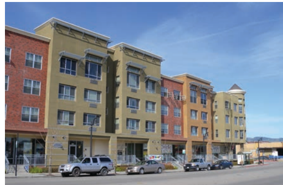
The facade is articulated to break the project down to smaller components and reduces bulk. (Guideline E-26 & 27)
