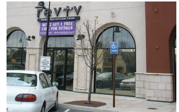
This project uses tile for the first three feet above the sidewalk level, which is highly durable and adds a decorative element to the ground floor design. (Guideline E-7)
