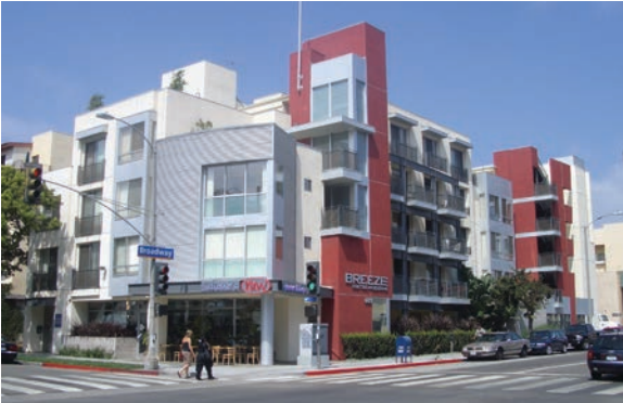
The building bulk is broken up through height recesses along the length of the building. (Guideline C-5)
