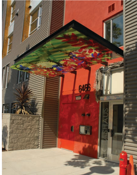
The special treatment of the awning highlights the entrance of the building. (Guideline D-8)
