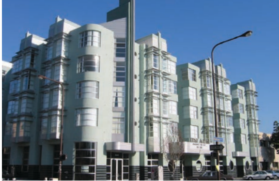
This project exhibits consistent design integrity, as the building components are in keeping with the Art Deco style. (Guideline E-1)
