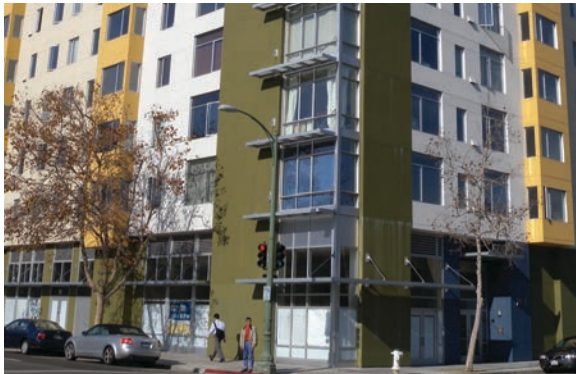
The green and yellow colors on this facade serve as accent colors, rather than being used for the entire facade. (Guideline E-15)
