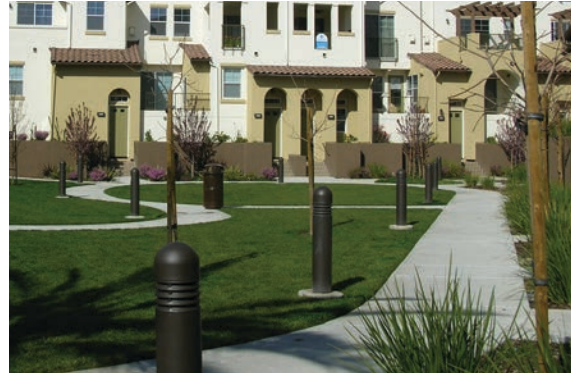
Provide landscaping within common open space areas. (Guideline J-3)
