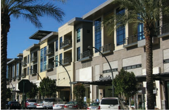
The building facade incorporates building projections, such as balconies, and recesses which enhance the design and articulation of the building. (Guideline E-27)
