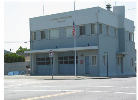
Alameda County fire station
