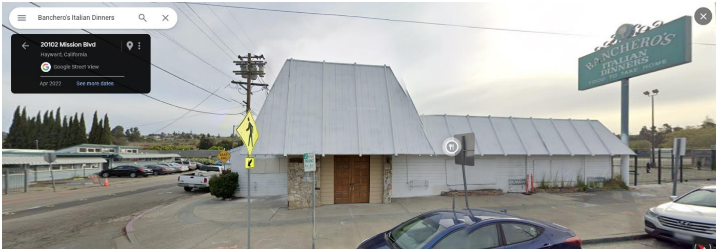
Figure B-1. The most recent Google imagery of 20102 Mission Boulevard (April 2022).
