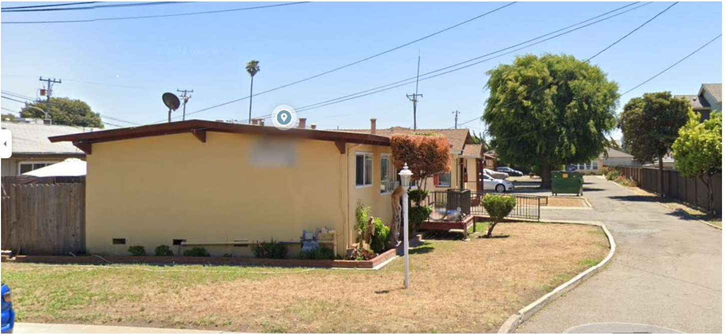
Figure B-34. Recent street imagery of parcel (2024).
