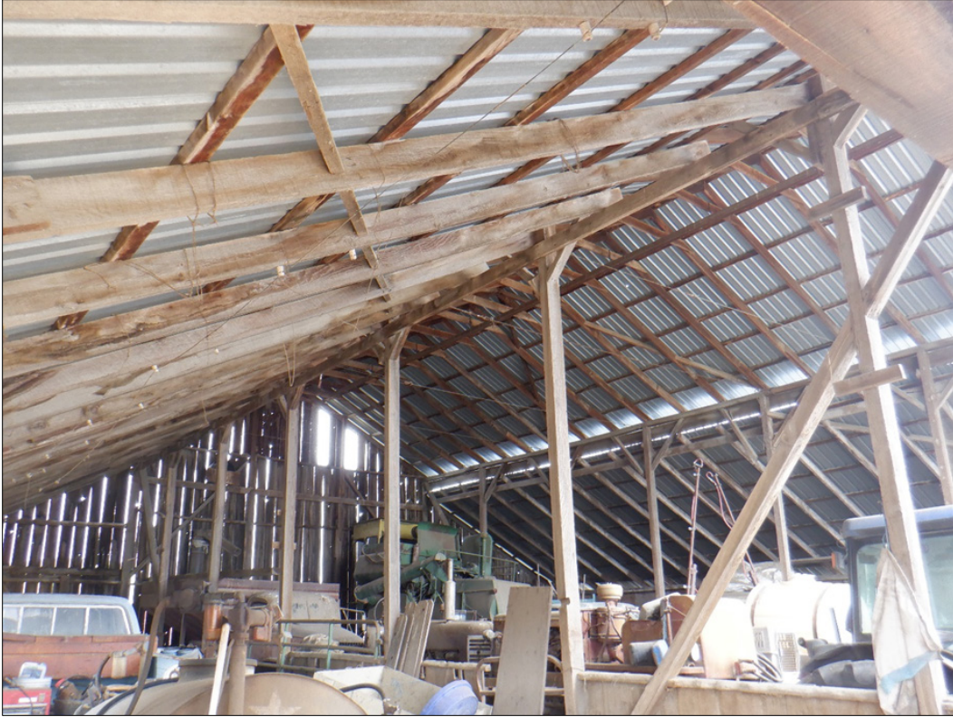
Figure 20. Barn interior, looking west
