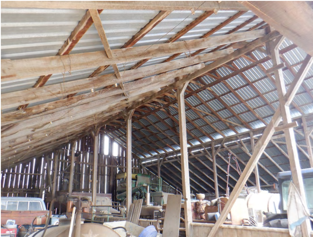
P5b. Description of Photo: Barn interior, looking west.
