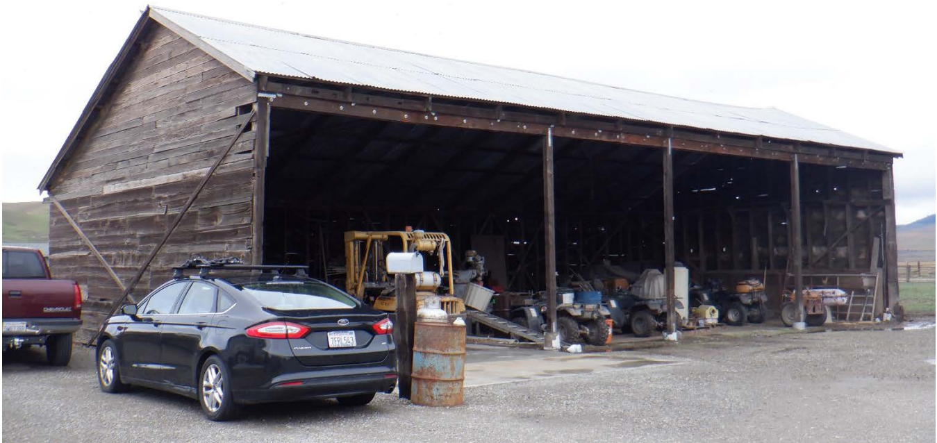
P5b. Description of Photo: Shed south and east façades, looking northwest.
