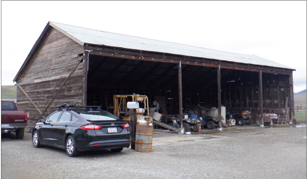
Figure 21. Shed south and east façades, looking northwest
