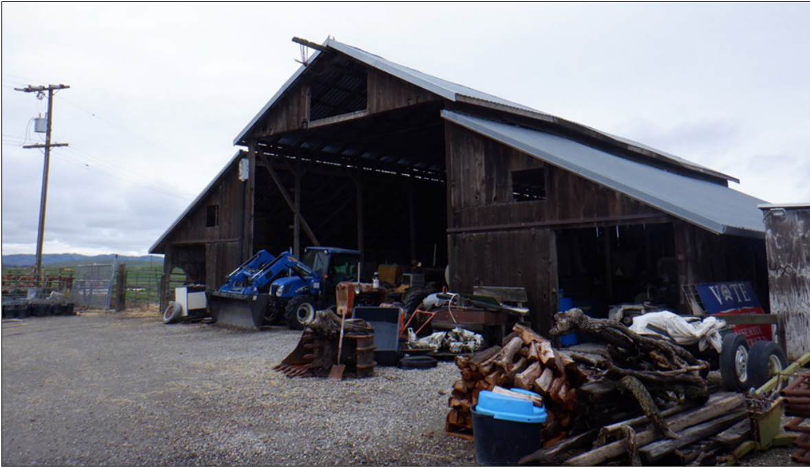
Figure 14. Barn east façade, looking southwest. Notice the large expanded opening and the protruding hay rail from the front gable
