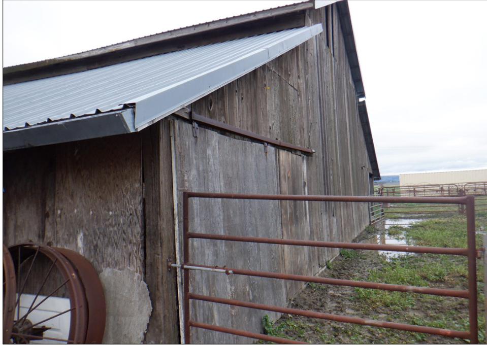
Figure 18. Barn west façade, looking southeast. Notice the plywood sliding barn door
