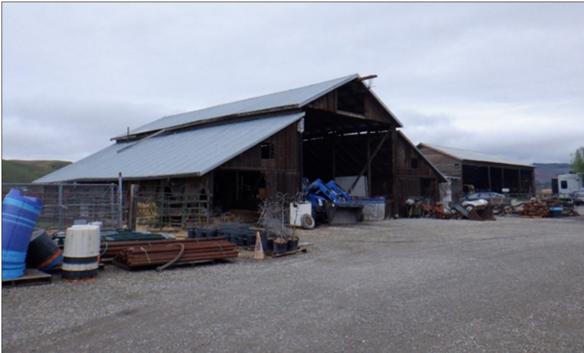
Figure 13. Historic post-and-beam vernacular barn and shed east and south facades, looking northwest from the gravel driveway
