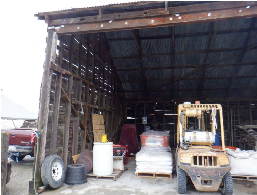
P5b. Description of Photo: Interior of shed with its post and beam construction, looking west. Notice the primary support beam above with metal brackets. An older support beam with mortise rests above the newer primary support beam. This beam most likely comes from an older structure which is a common feature of vernacular ranching structures.
