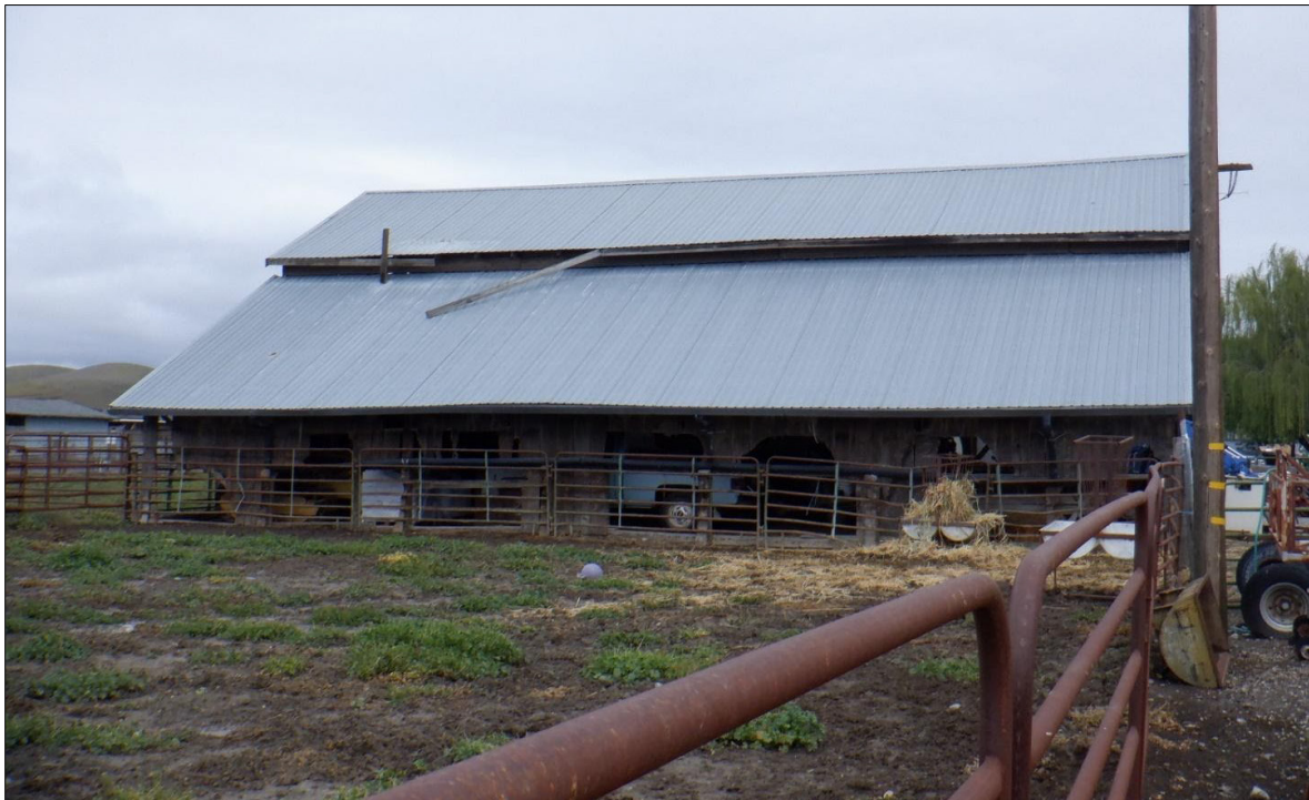
Figure 15. Barn south façade with openings, possibly for cattle, looking north
