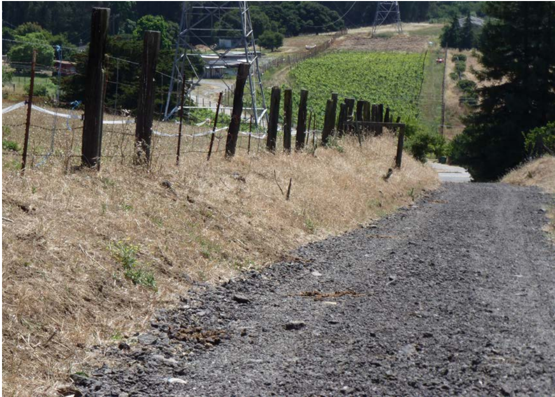
Figure 3.17: Looking west, downslope along existing dirt access road; Fairview Avenue is at foot of slope; PG&E parcel is on the left
