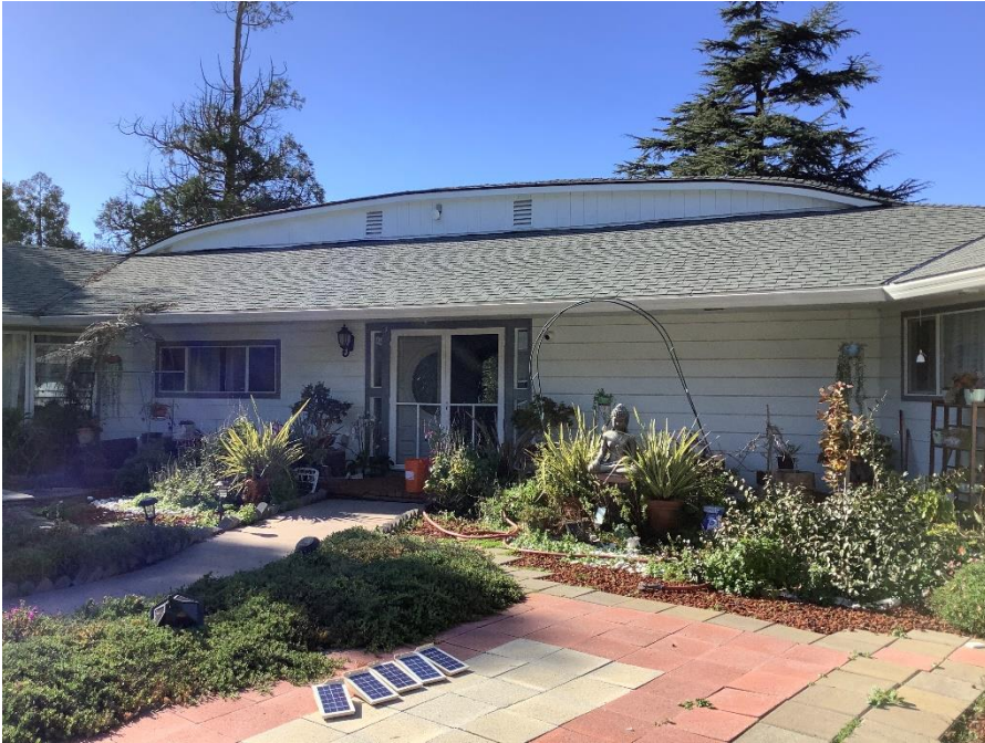
Figure 11. View of primary (east) façade of ancillary residence, looking west. January 20, 2023.
