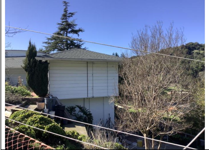
Photo 10. Northeast facade of north wing, facing southwest.
