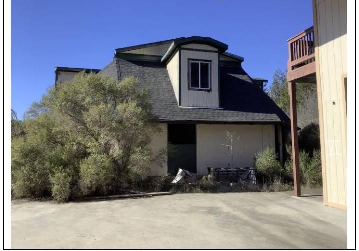
Photo 22. East facade from open-air garage entrance, facing west.
