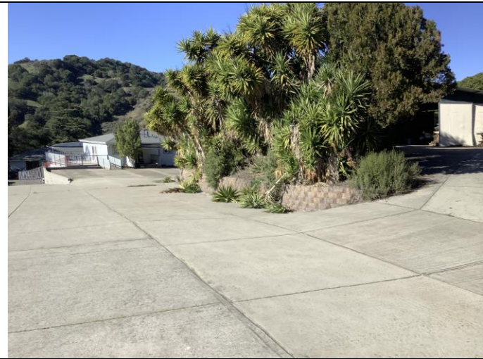
Photo 35. Lower grouping from long driveway, facing northwest. View includes middle horse barn, small residence with garage, and main residence.
