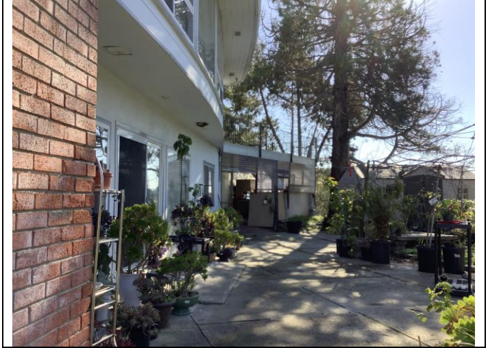
Photo 14. Main residence, south wing and part of west facade, facing southeast.
