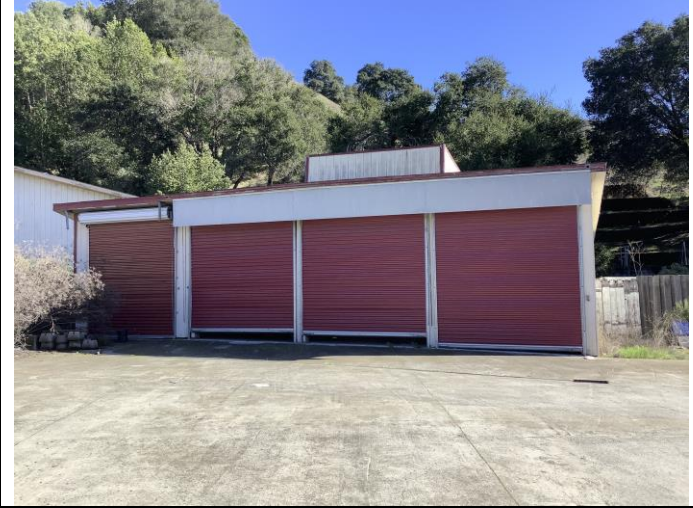
Photo 45. Garage, facing east.
