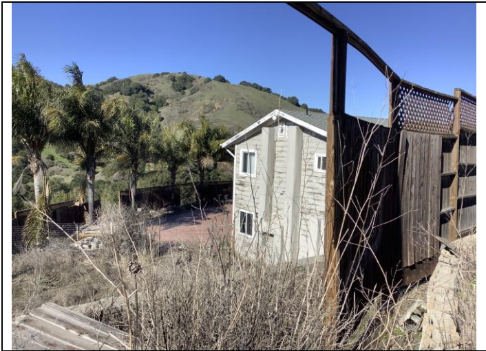
Photo 32. South facade of ancillary residence (Building 4), facing northwest.
