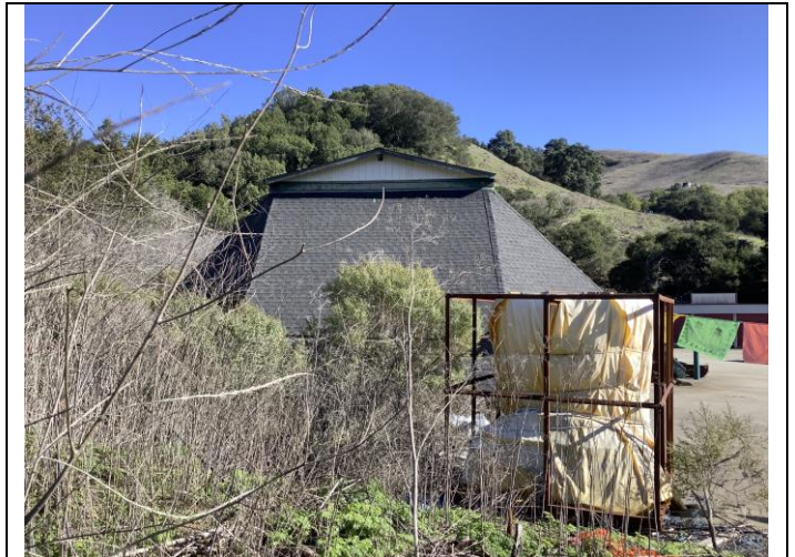
Photo 24. West facade of barn from paddock, facing east.
