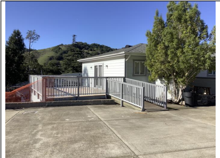
Photo 20. Garage and residence east and south facades, detail of deck, facing northwest.
