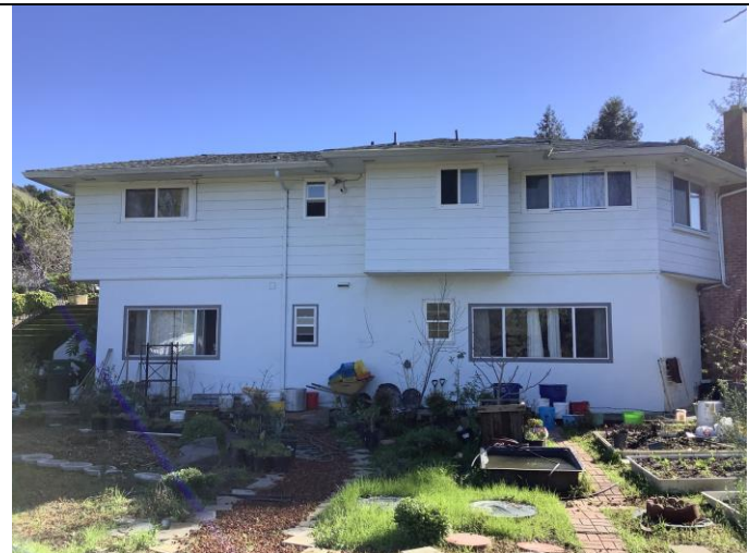
Photo 11. West facade of north wing, facing southeast.
