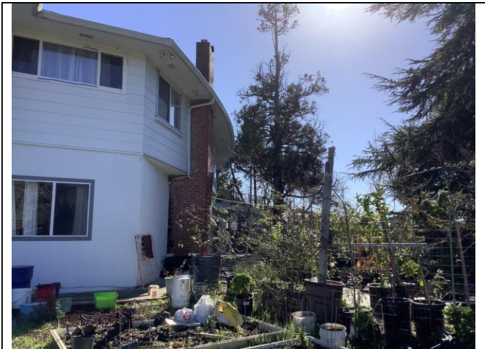
Photo 12. Main residence, west facade with north wing, facing southeast.
