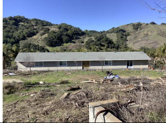
Photo 33. Ancillary residence from garden, facing west.
