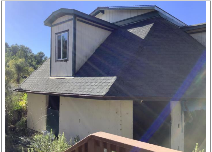
Photo 28. Barn from second floor of open-air garage (Building 9), east facade, facing southwest.
