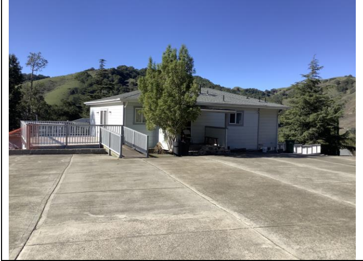
Photo 18. Garage and residence east and south facades, facing northwest.
