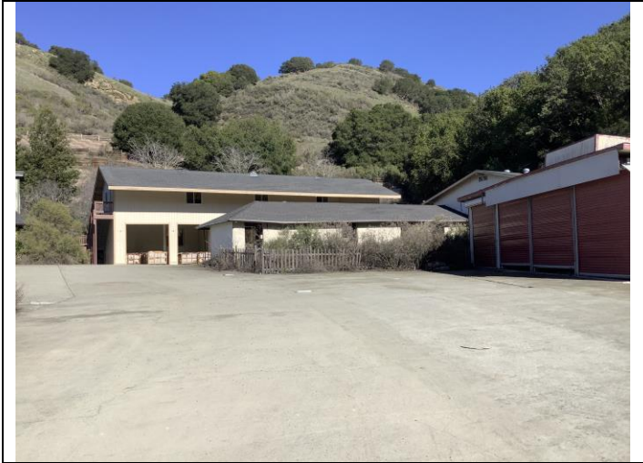
Photo 40. Upper grouping including open-air garage, storage barn, garage, and hillside, facing north.
