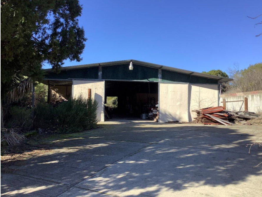
Figure 13. View looking northwest toward middle barn. January 20, 2023.
