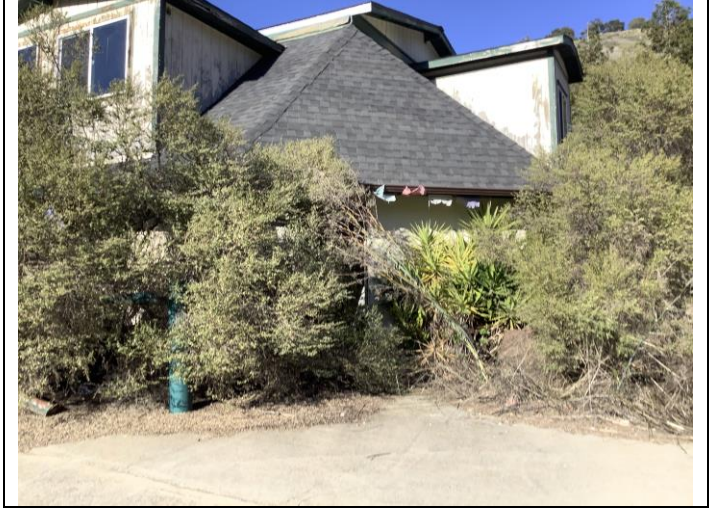
Photo 26. Southeast corner of barn, facing northwest.
