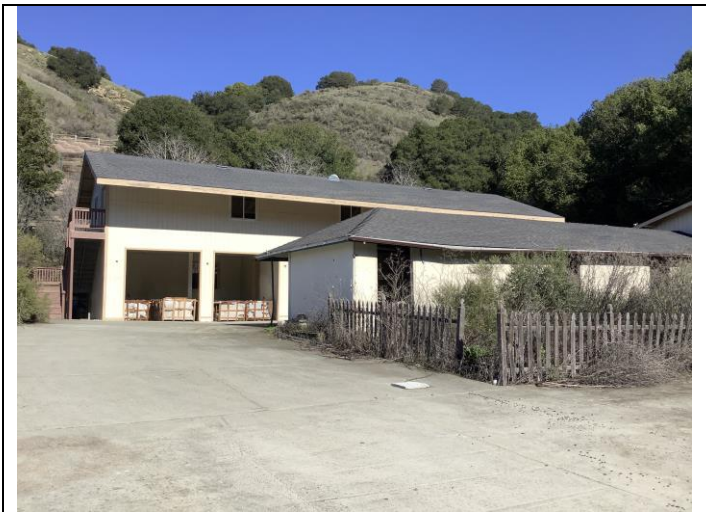
Photo 48. Open-air garage, facing northeast.
