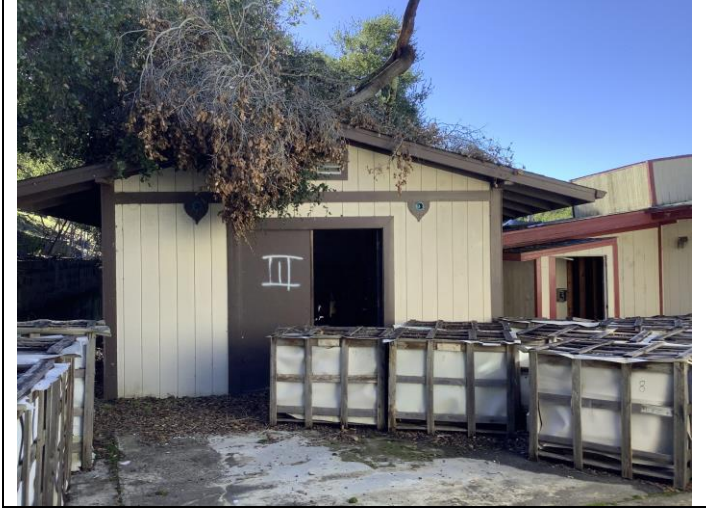
Photo 46. Rear garage storage building, facing south.
