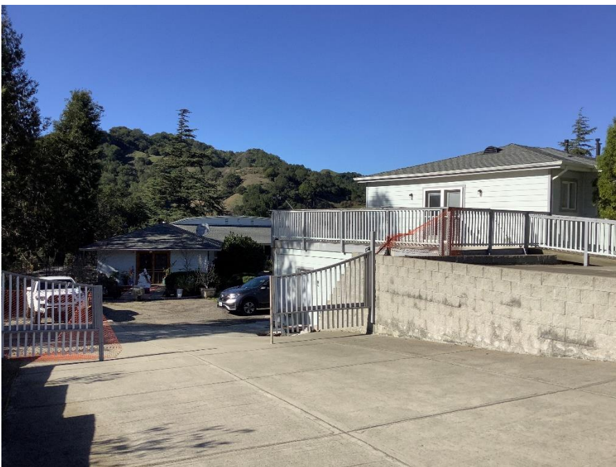
Figure 12. View to west of garage and residence. January 20, 2023.
