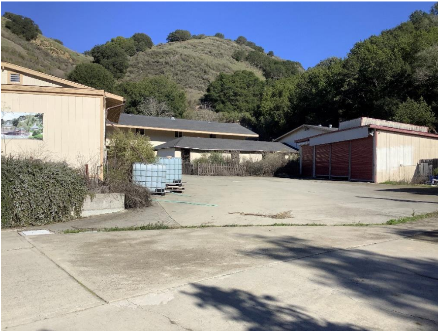
Figure 16. View northeast of upper grouping including barn, open air garage, storage barn, red door garage, and small manufactured home. January 20, 2023.
