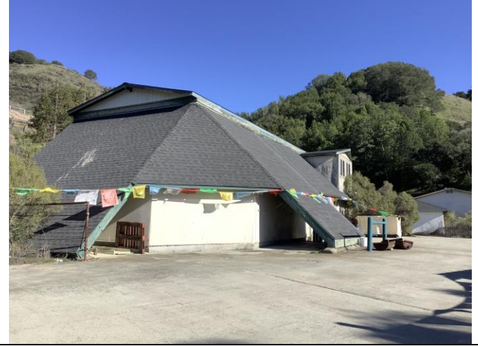
Photo 25. Southwest corner of barn from paddock, facing southeast.
