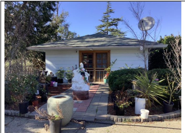
Photo 8. Southeast facade of the south wing of main residence, facing west.
