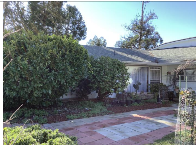
Photo 7. South wing, facing southeast.
