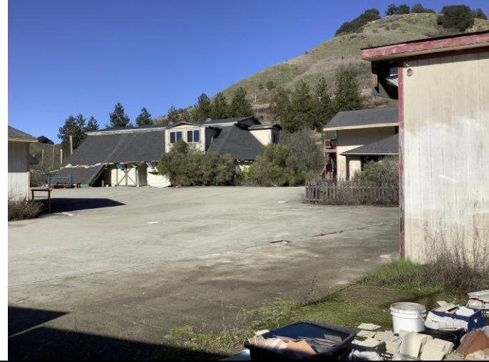
Photo 41. Upper grouping including barn, open-air garage, storage barn, garage, and small manufactured home, facing northwest.
