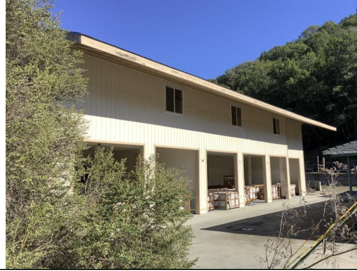
Photo 49. Primary facade of open-air garage, facing northeast.
