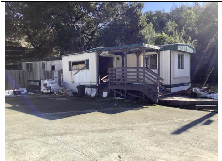
Photo 44. Mobile home entrance, facing southwest.
