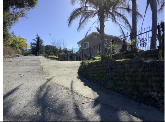
Photo 29. Ancillary residence (Building 4), north facade from steep driveway, facing southeast.
