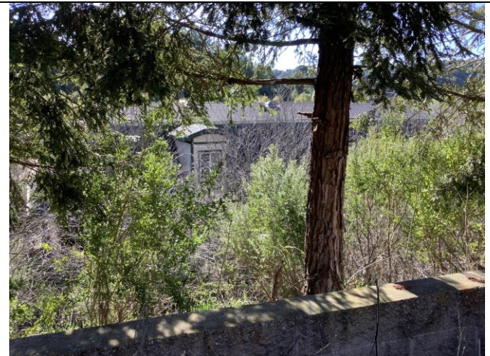
Photo 23. North facade of barn from rear retaining wall, through large brush, facing south.
