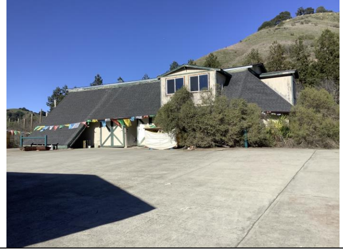
Photo 21. South facade of barn, facing north.
