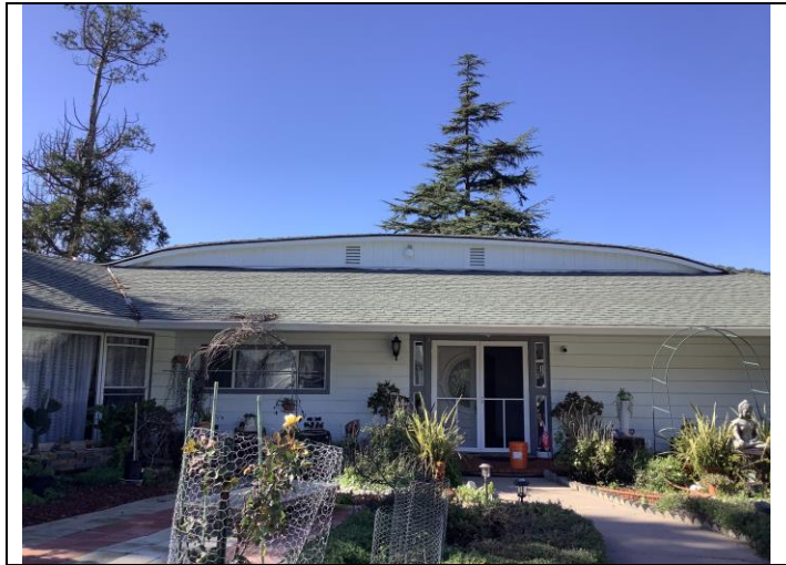
Photo 4. Central entry court, facing west.
