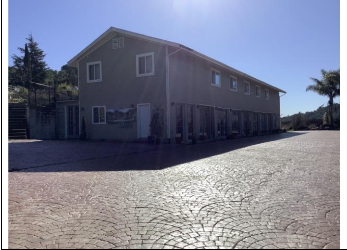
Photo 30. North facade and east facades of ancillary residence (Building 4), facing southeast.
