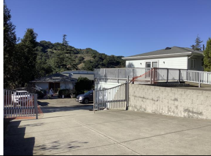
Photo 17. Garage and residence, building with main residence in background, facing west.
