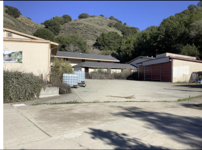
Photo 39. Upper grouping including barn, open-air garage, storage barn, garage, and small manufactured home, facing northeast.
