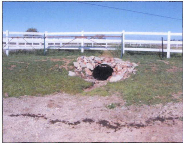
Picture 6: Culvert at the western end of the project site where ED 5 terminates and flows under Greenville Road.
