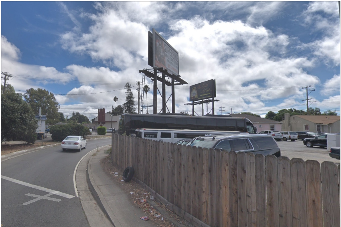
Sign #2767 E. Lewelling Blvd 160 ft W/O Mission Blvd
