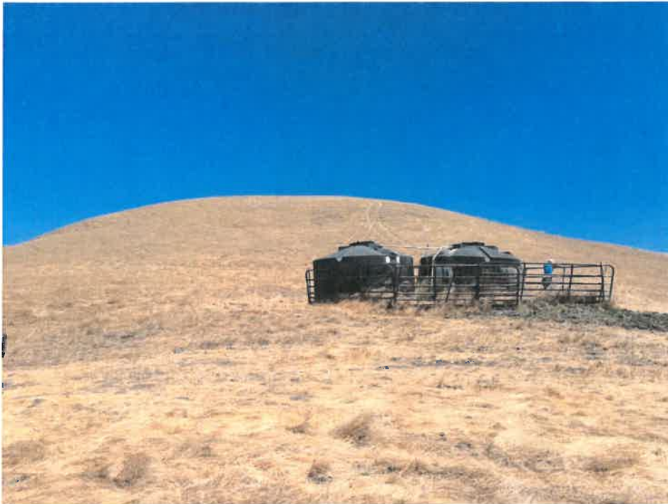
Photo 2. Water tanks located near the top of the property
