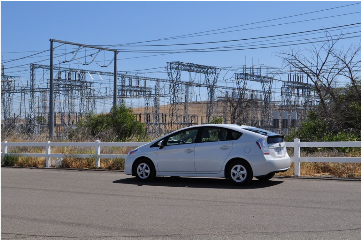
4. Midway Substation from Patterson Pass Road looking east.
