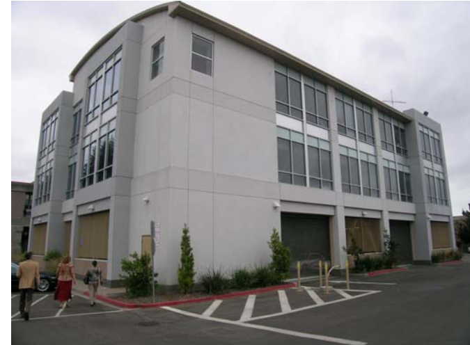
Public Works Agency Building (new addition) at 399 Elmhurst, Hayward
