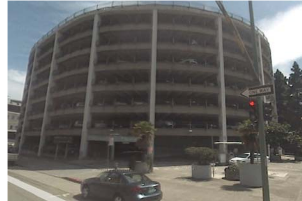
ALCO Park Parking Garage, Oakland
