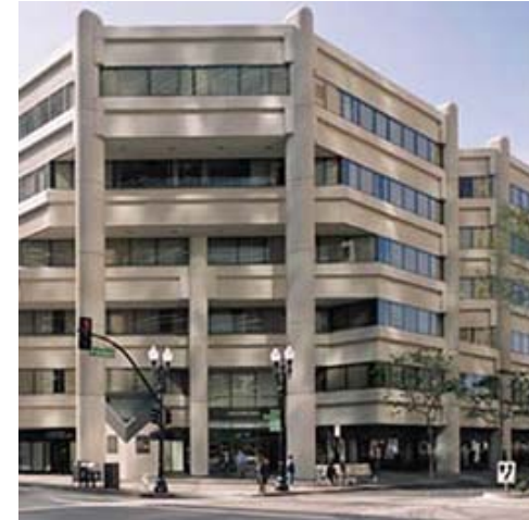
Public Health Department Building At 1000 Broadway, Oakland
