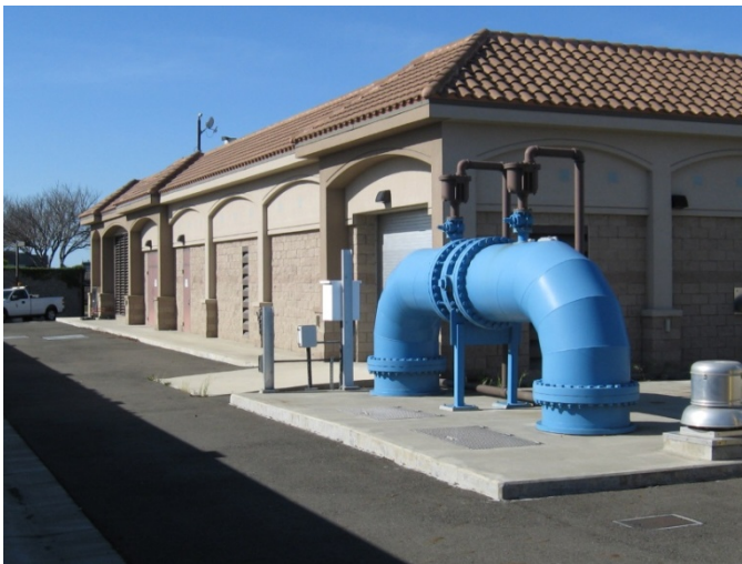
Skywest Pump Station
