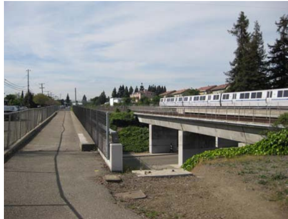
The Whitman Street overcrossing provides an existing grade-separated pedestrian and bicycle crossing of Carlos Bee Boulevard immediately parallel to the Oakland Subdivision. Other arterial grade separations along the corridor do not have such existing facilities.
