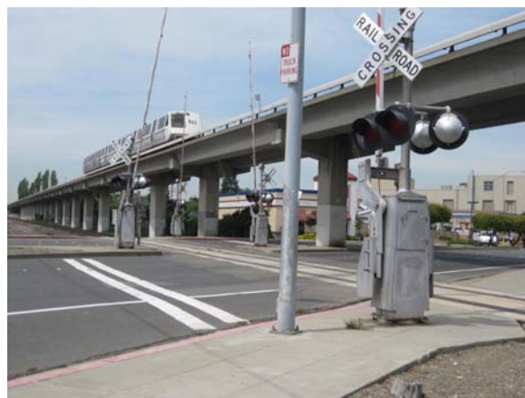
The existing at-grade rail crossing at Hesperian Boulevard in Oakland is 375 feet from the nearest existing controlled intersection at Ruth Court
