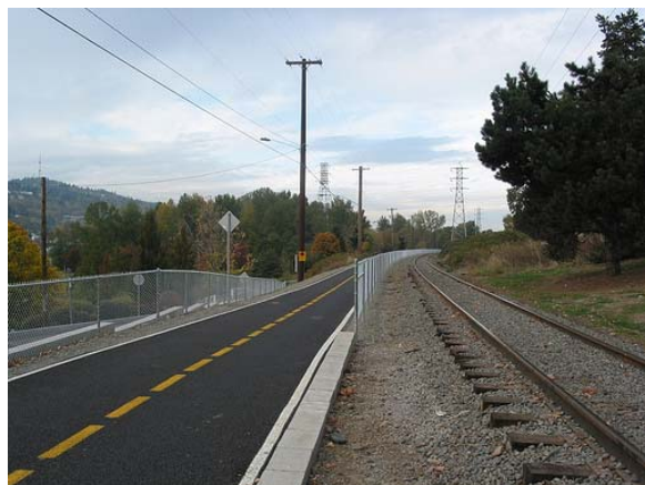
The Springwater rail-with-trail in Portland, Oregon is setback less than 10 feet from the centerline of the adjacent low-use and low-speed freight spur. A four foot chain link fence provides separation.
