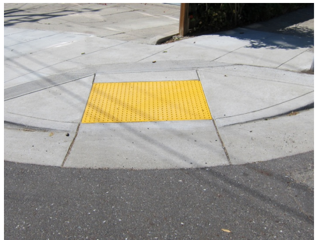
Figure 4-3: Curb ramp with detectable warning strip
