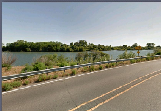
Center Line Rumble Strip
