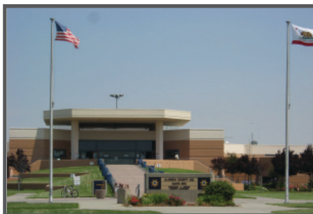
Energy and water efficiency are a priority at the 24/7 Santa Rita Jail.
